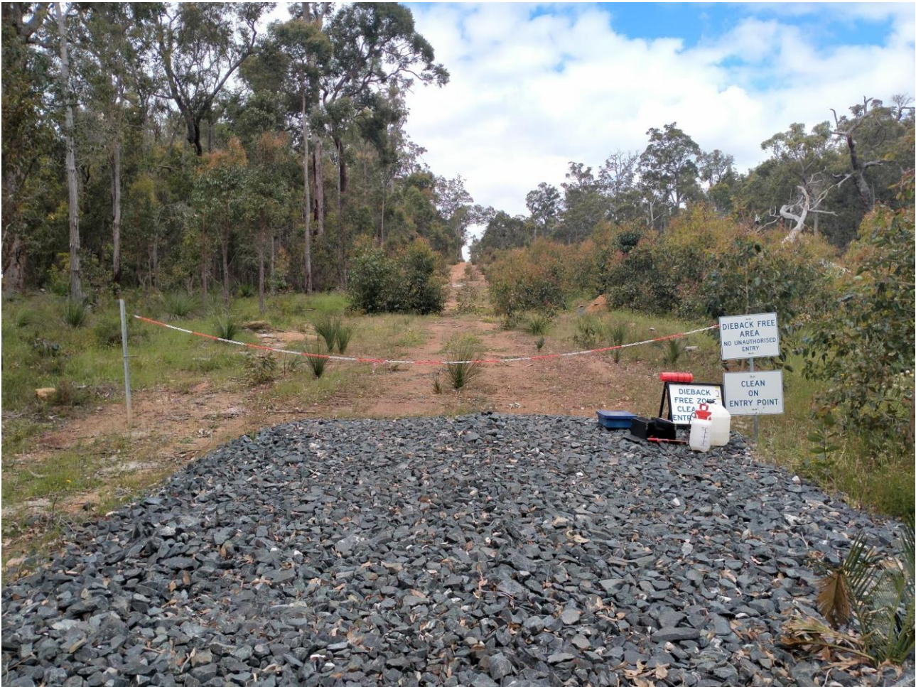
Figure 5: CoE Point established, with signage, barricading, gravel-lined washdown bay, cleaning solution and sign in register
